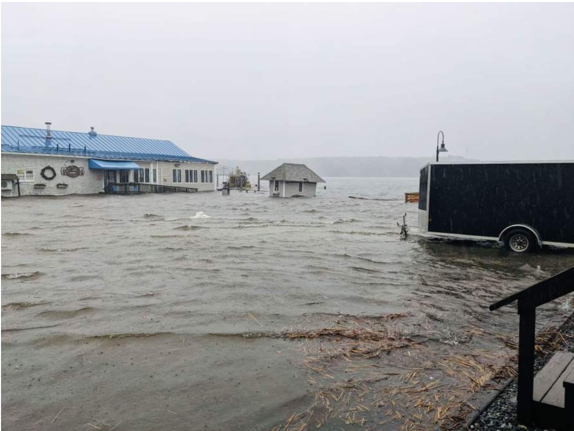
Photo 1 - December 23, 2022 Flooding near Commercial Street
