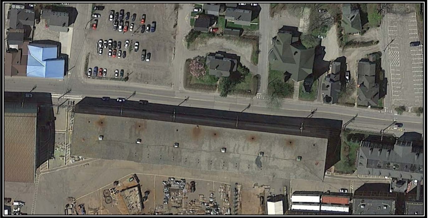
Figure 7: Site #3 - Washington Street near Bath Iron Works
