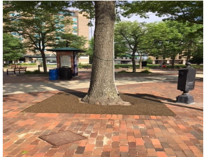
Porous pavement expands tree root access to water
